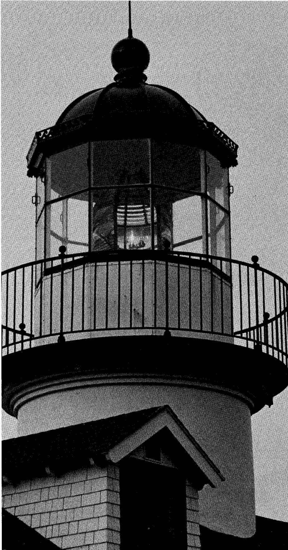
The lantern room of the Point Pinos Lighthouse.
