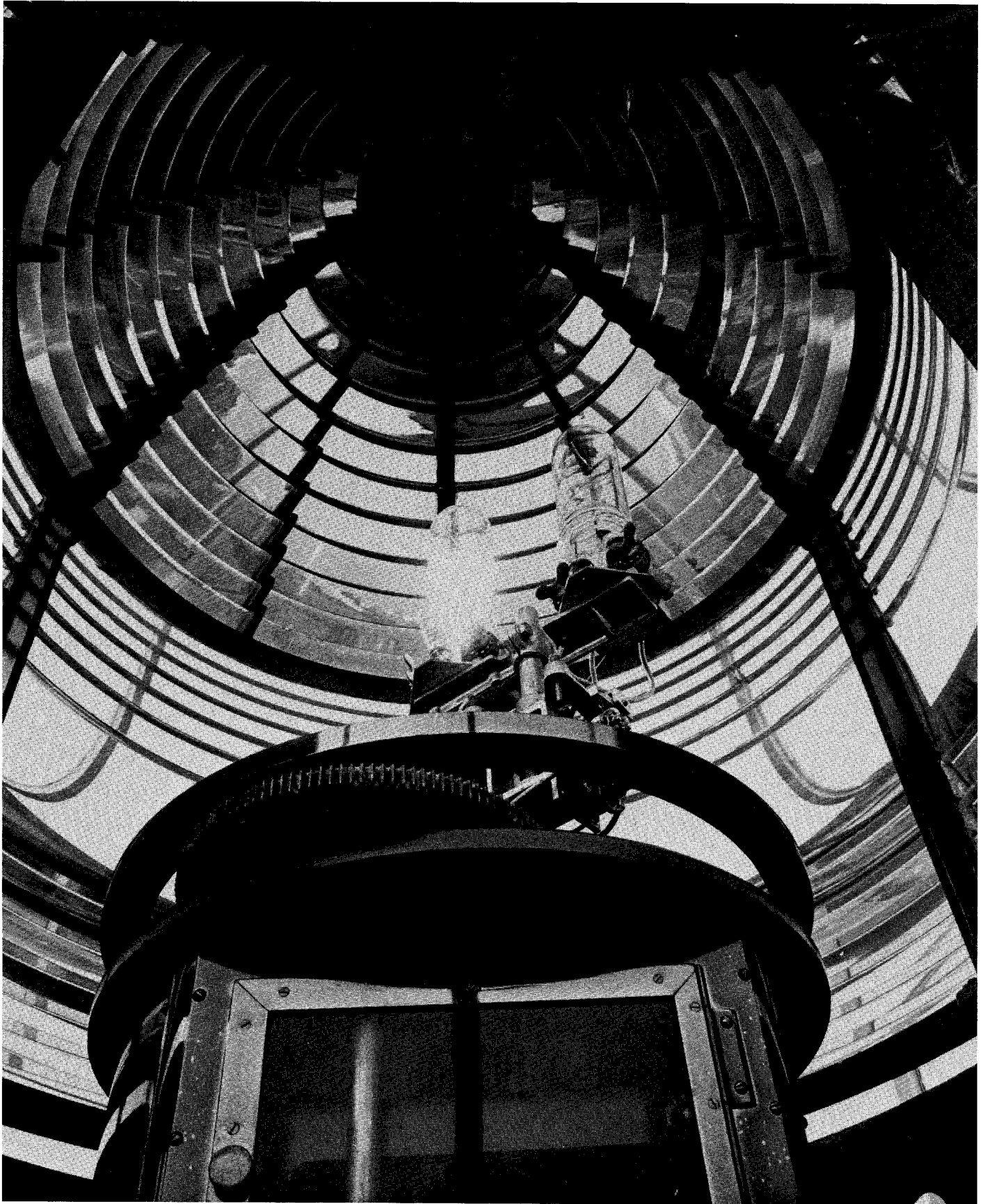
The original 3RD Order Fresnel lens that Emily Fish polished is still in operation. In later years a clockworks was installed that rotated a brass panel ("eclipser") which gave the light a flashing characteristic.
